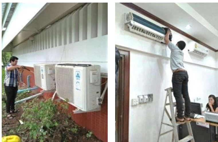
Figure 4 Cleaning air conditioner to reduce energy consumption
