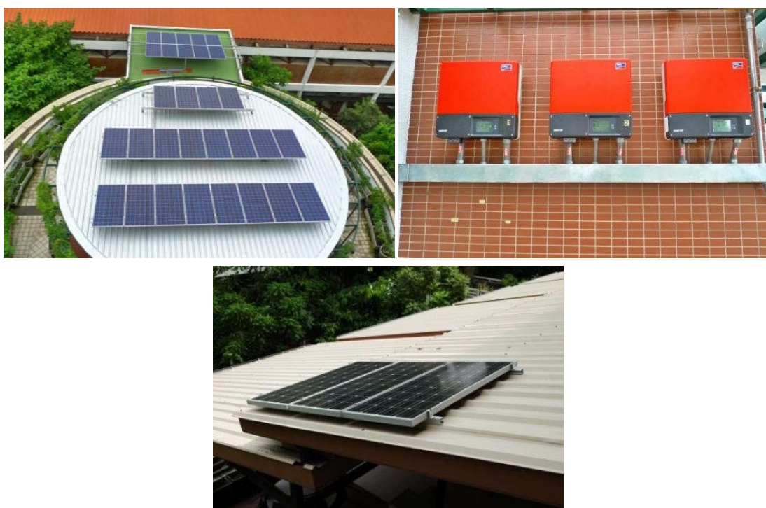
Solar Cell Panels 9 Kilowatts.
